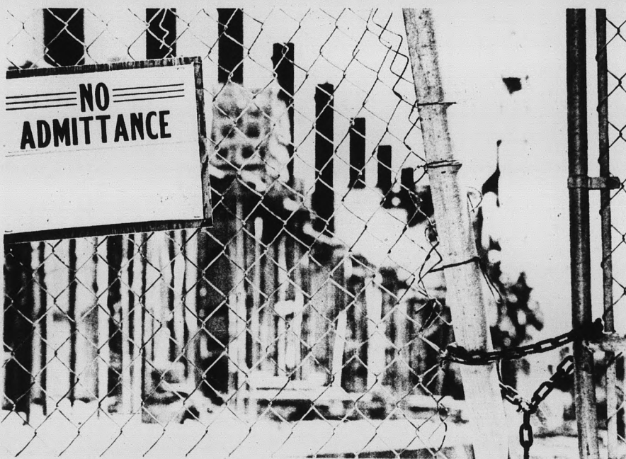
Library construct area: a ghost town during the strike
