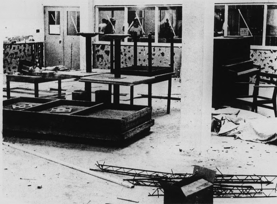
Clancy's in the MU basement under goes a remodeling
