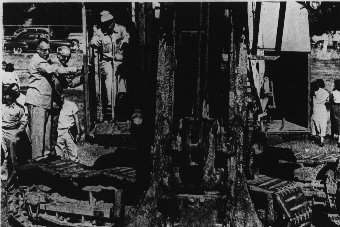
GROUND BREAKING — The first scoop of earth moved at the ground breaking of the MU in 1955. Standing on the shovel was College President Grady Gammage, and Charles Stauffer, former
