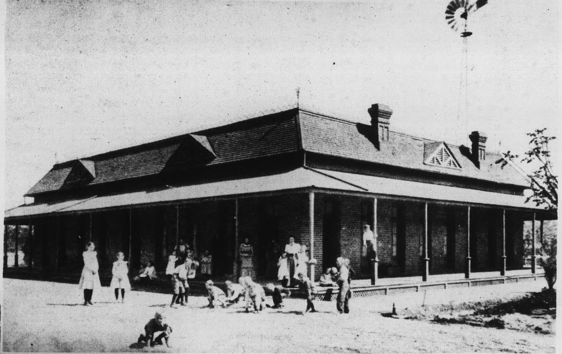
FIRST NORMAL SCHOOL BUILDING —This proud structure contained the classes in the school's opening year, 1886. That first year the school consisted of 33 students and professor-principal Hiram Bradford. The four-classroom, one-story building cost $7,000, a small amount compared to the $3.6 million needed to construct the new library.
