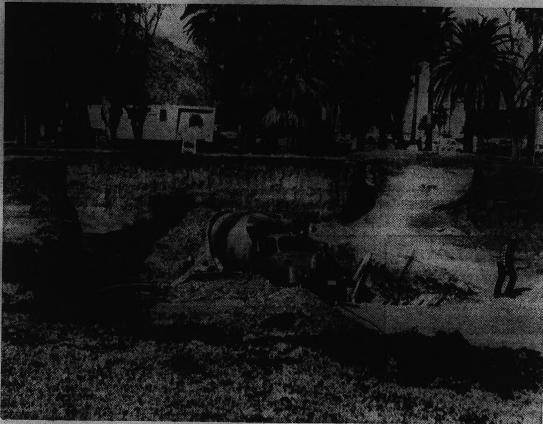
TODAY A HOLE — But tomorrow, the six-story Language Arts building (below) will rise from the pit that now enhances the old park. (State Press Photo by Larry Ward)
