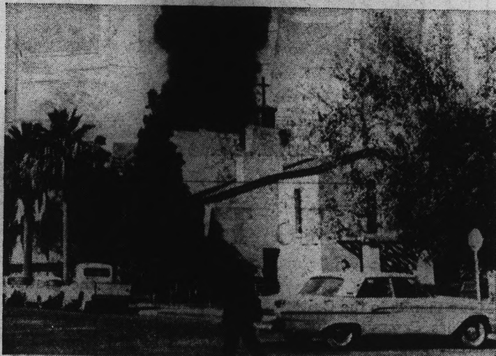
HOLY SMOKE? — Not really, it just appears that way as smoke billows skyward behind Danforth Chapel during a fire that totally destroyed Sportcraft Trailer Mfg. Co., Inc. (Photo by Ed Ryan)
