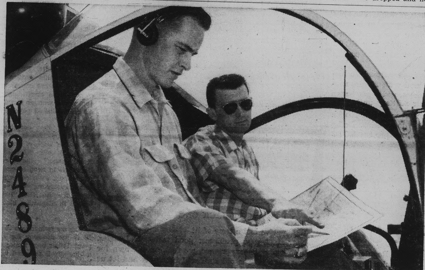
Telephone engineer Bill Pigott, left, and helicopter pilot plan aerial exploration for microwave tower sites.
