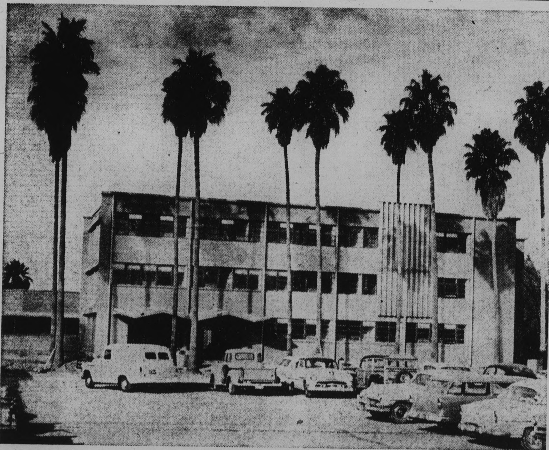
NEW LIFE-SCIENCES CENTER . . . will receive its first occupants during summer sessions. Complete occupation of the $972,800 structure is expected to take place in September.
