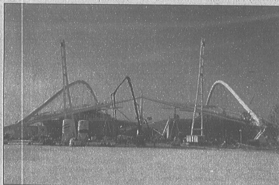
Construction of the Olympic Stadium
