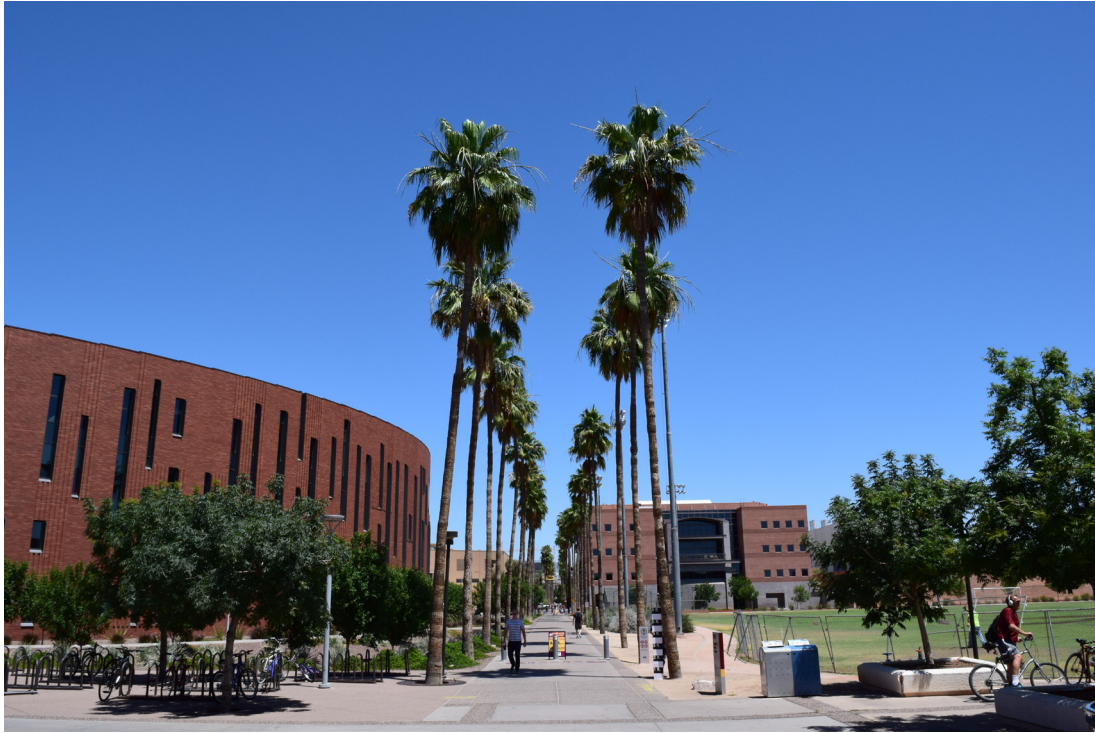
Figure 11. South end of Palm Walk, May 2016, view to north. McCord Hall is to left (photo by Paul Molter, ASU).
