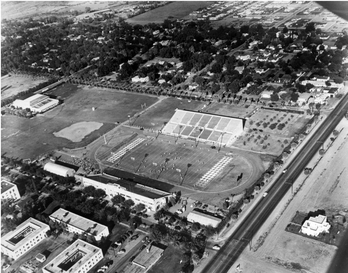
Figure 9. 1950 aerial photograph. Rows of palms are seen in distance, along Normal Street, behind bleachers of athletic field. U.S. Highway 60 (Apache Boulevard) is to lower right (Courtesy University Archives, Arizona State University Libraries).
