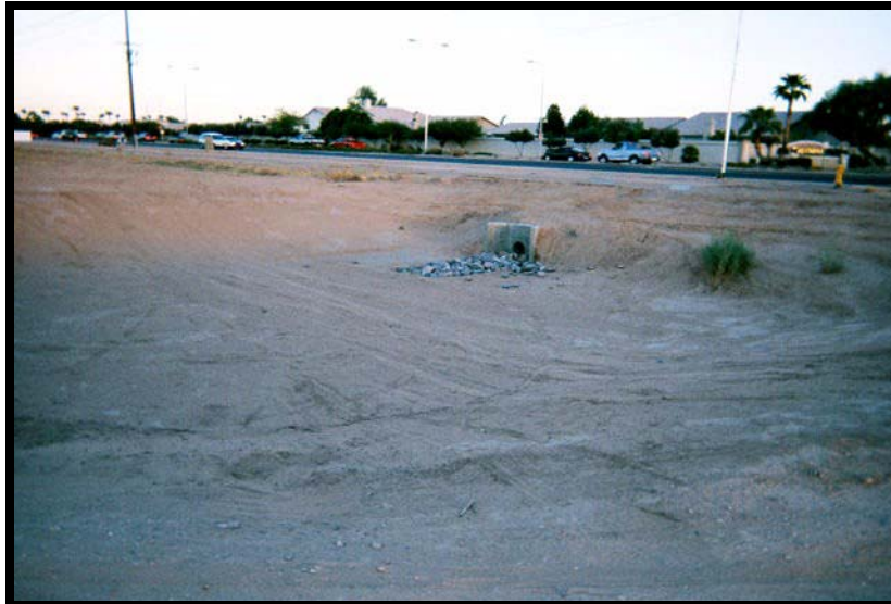
Temporary sediment basin with outlet protection.
