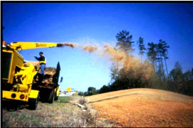
Mechanical chipper application of mulching
