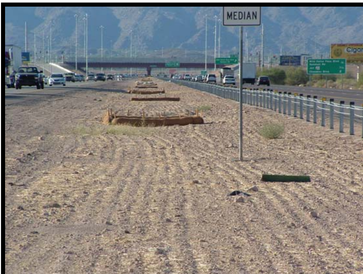
Use of an organic filter barrier in the highway median.
