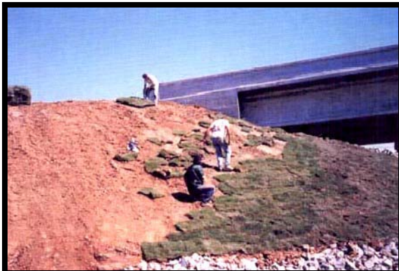
Applying sod to a slope
