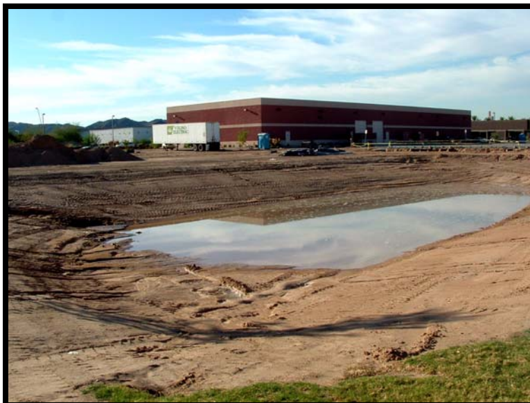
Temporary sediment basins provide stormwater storage during the construction process.
