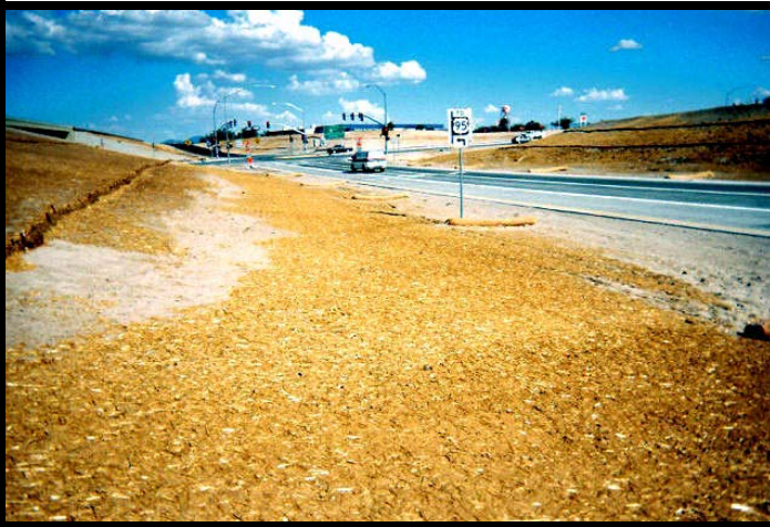
Mulching protects exposed areas and seeding for revegetation.
