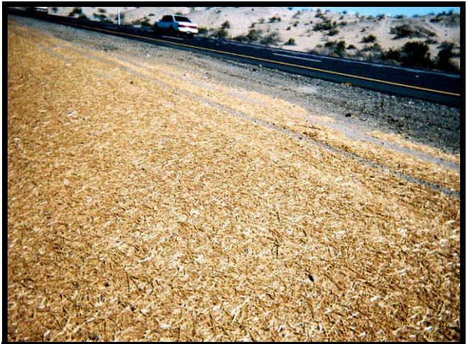
Straw mulching along the shoulder of a highway.
