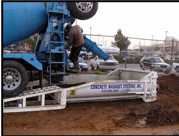
Concrete washout container.
