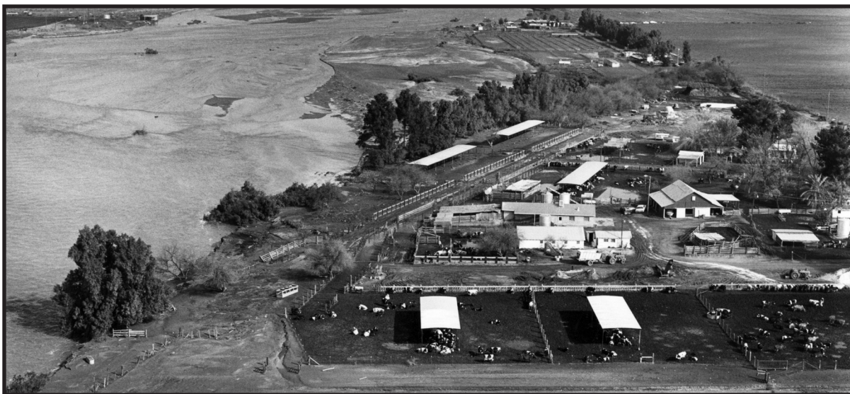
Agua Fria River and McDowell Road, Avondale, February 22, 1980
