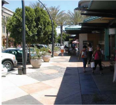
Photo 1.4.1 High Albedo Materials
