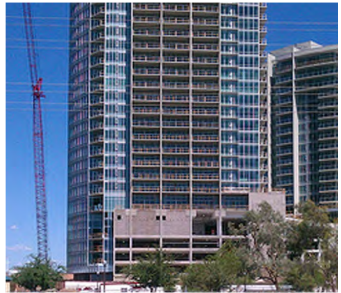
Encore on Farmer Street between 6th and 7th Streets, Tempe Arizona, offers low-income housing for seniors 55 and older. Source: http://www.raillife.com
