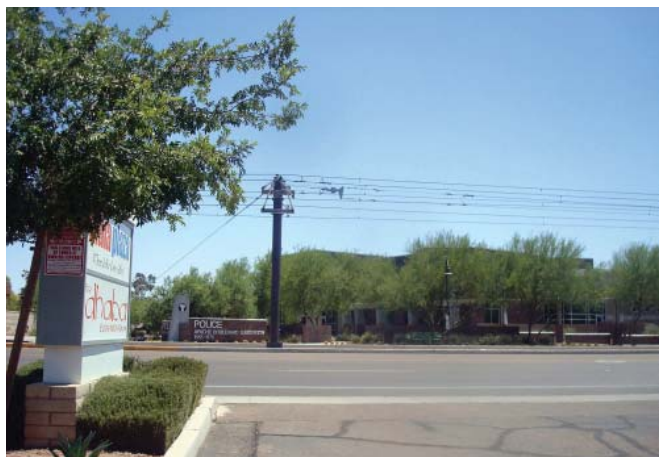
Apache Boulevard Police Substation
