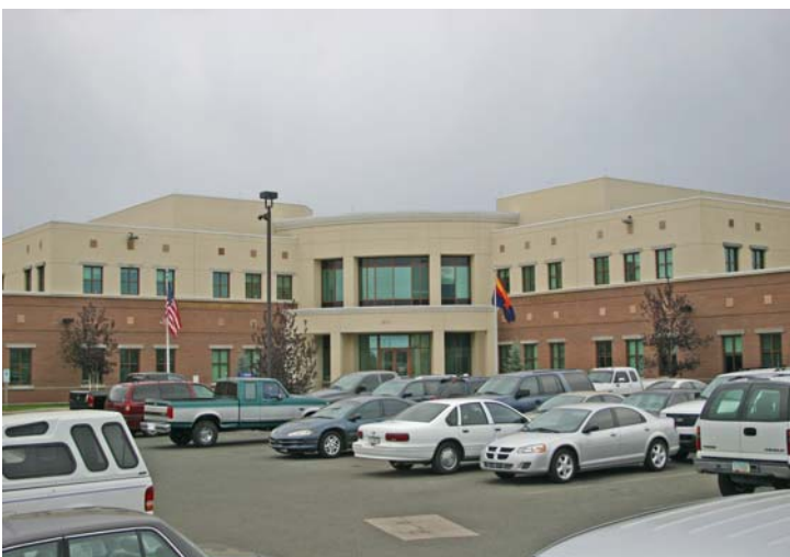
Law Enforcement Administration Facility
