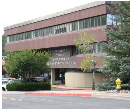
Administrative Center - Home to Finance
