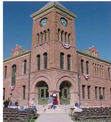
Coconino County Courthouse - July 2002
