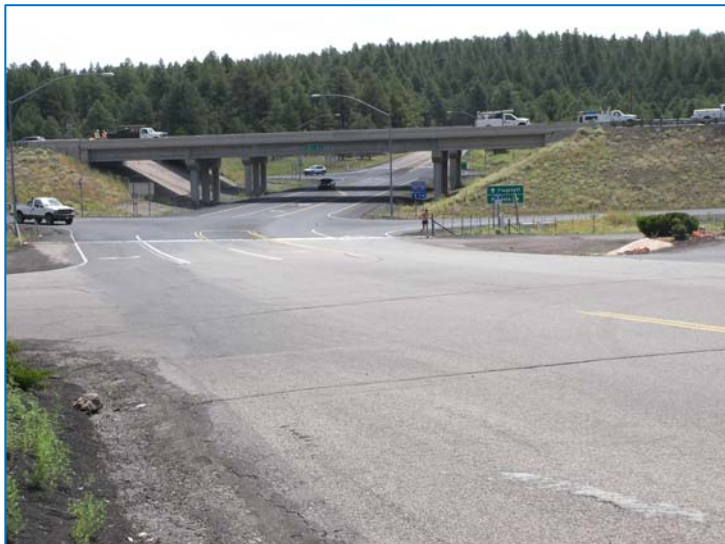
Picture of I-17 interchange looking east. Source: Kimley-Horn and Associates, Inc.
