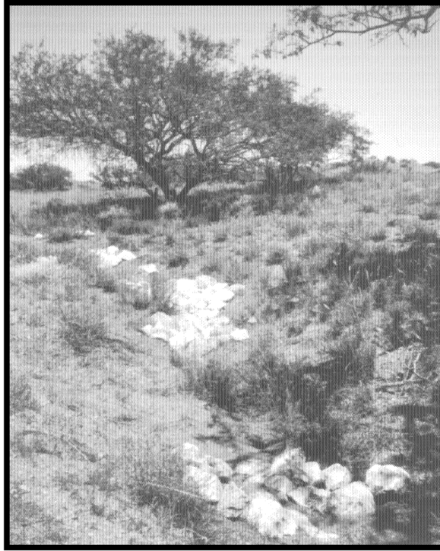
Figure 15. Headcut treatments in Oak Tree Canyon designed to decrease flow velocity and energy. 97-034WPF
