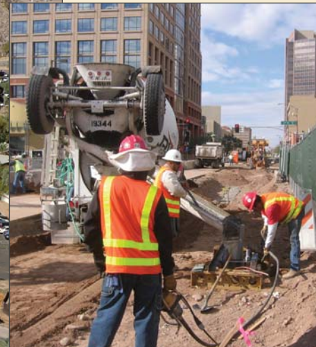
Guideway installation on Washington St.
