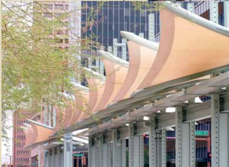
The station shade structure is complete at Central Station/First Avenue.
