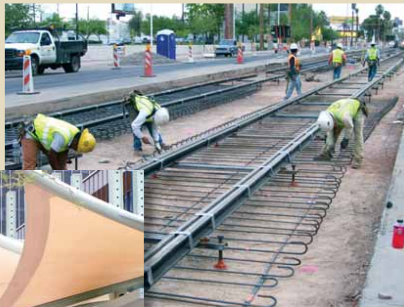
Guideway installation on Central Avenue near Indian School Road.
