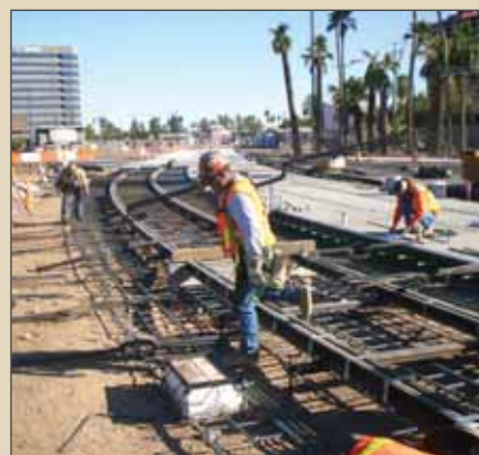
Rebar placed for the guideway on Camelback Road near Central Avenue Acero en la vía de guiado (guideway) sobre Camelback Road cerca de Central Avenue
