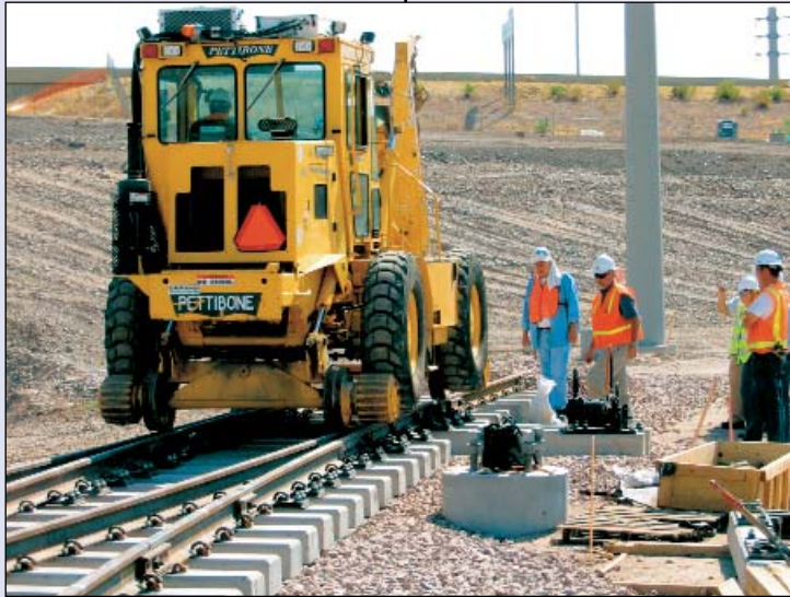
The first tracks are laid at the Maintenance and Storage Facility.
