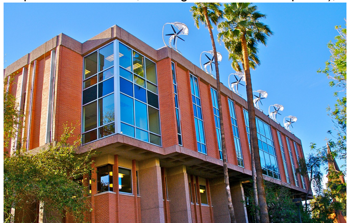
Wind turbines and solar panels atop the Global Institute of Sustainability generate up to 25 kW of electricity for the Tempe campus.
