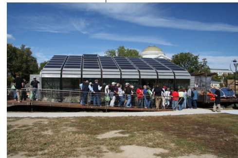
UA/AzRISE SEED[pod] Solar Decathlon House on the Mall in Washington, DC, one of 20 entries in the DOE competition, October 8-18, 2009
