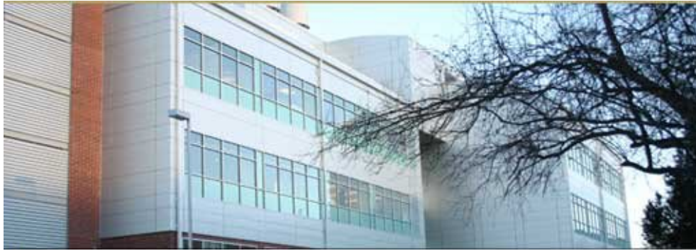
New Lab Building – equipment enhanced
