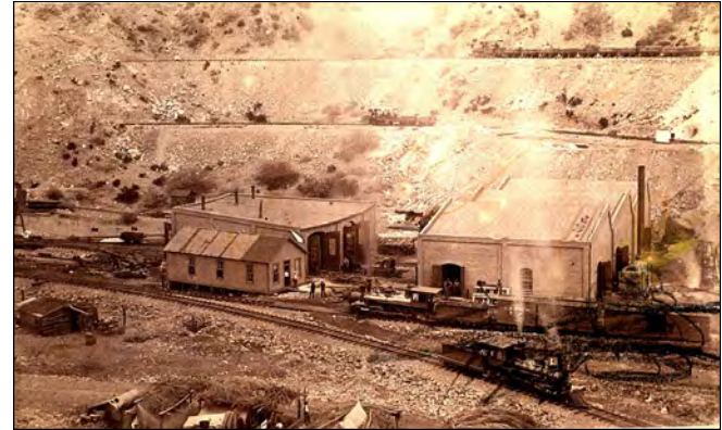
Railroad mine siding at the mine in Morenci, Arizona (Photo courtesy of Arizona State Library, Archives and Public Records, History and Archives Division, Phoenix, #94-2009)
