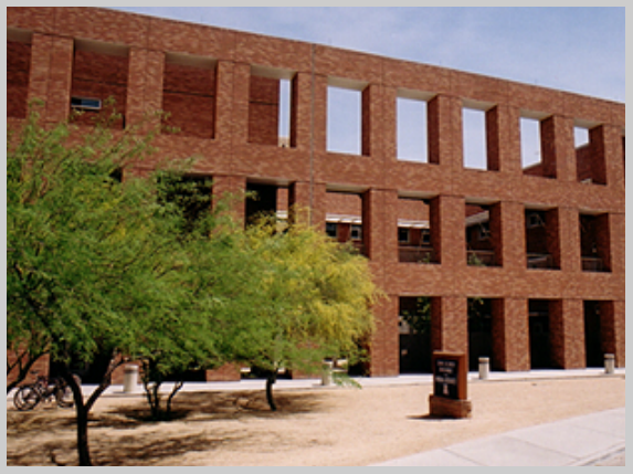
UA Dennis Deconcini Environment and Natural Resources Building (Photo courtesy of the University of Arizona)
