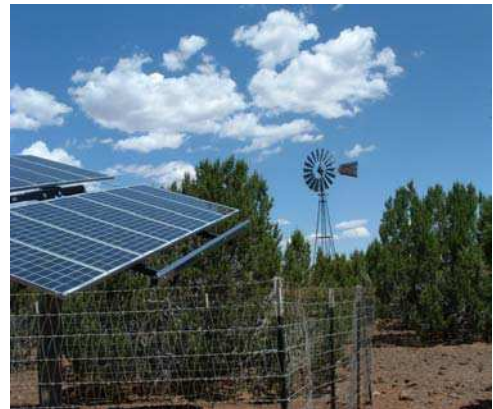
A LCCGP grantee in northern Arizona addressed water needs by installing a solar-powered pump on an existing well and providing additional water sources to wildlife, as well as livestock.
