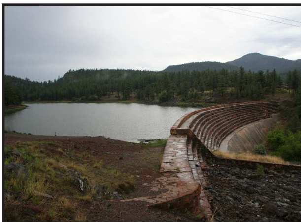
Santa Fe Reservoir, City of Williams. City of Williams historically relied on surface water stored in five small reservoirs. Since 1999, the city has drilled four wells to supplement surface water supplies.
