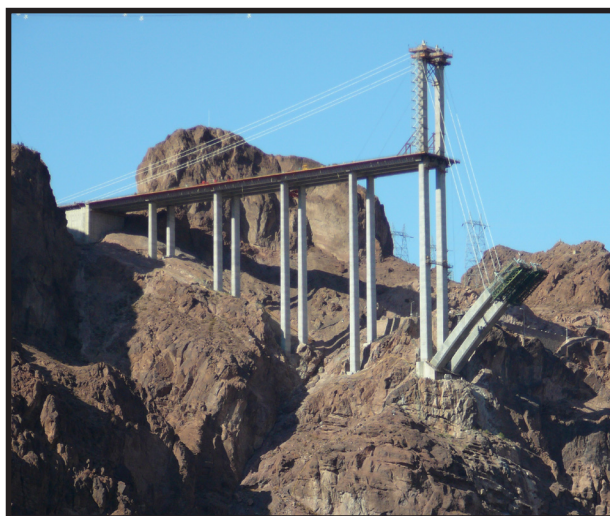
Hoover Dam bypass bridge under construction. There is concern in the planning area about large master-planned communities planned as a result of completion (2010) of the bypass bridge.
