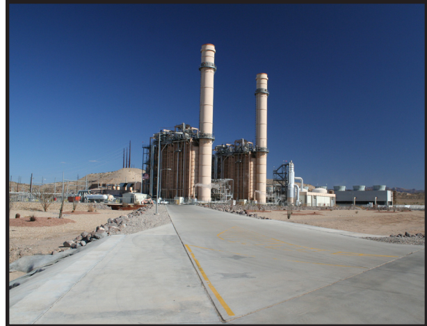
South Point power plant, Lake Mohave Basin.
