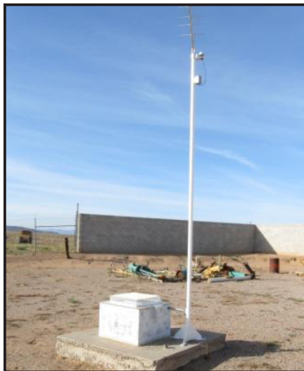
Automated Groundwater Monitoring Site in the Hualapai Valley Basin.
