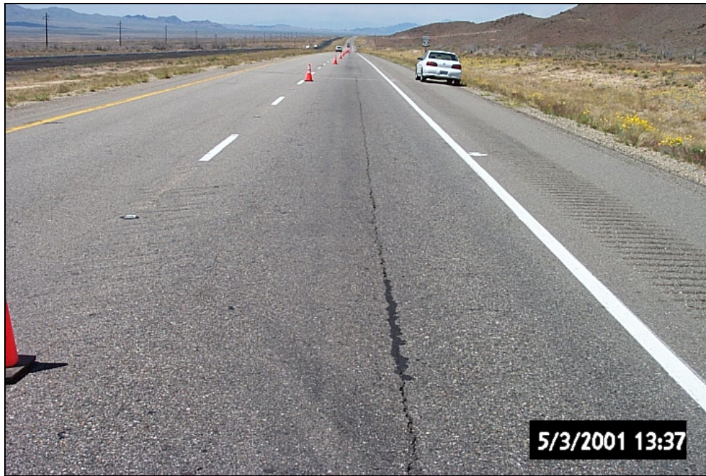
Figure 10. Photograph of paving seam.
