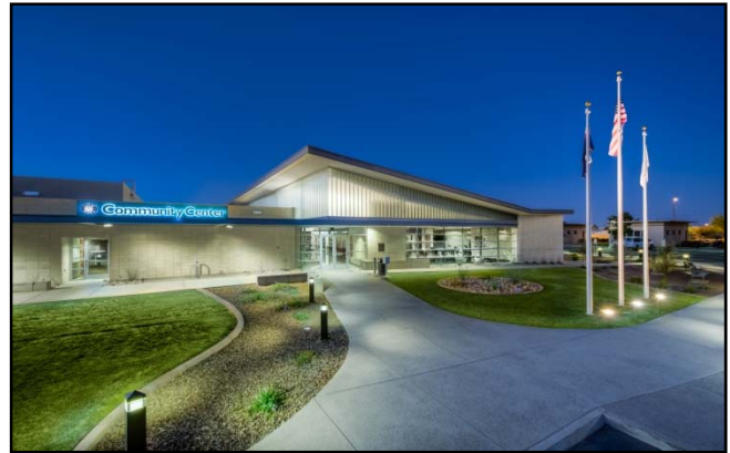
The Community Center in Old Town Peoria was recently remodeled and expanded.
