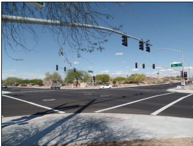
Deer Valley Road Improvements
