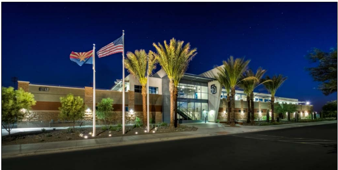
The San Diego Padres' newly renovated clubhouse
