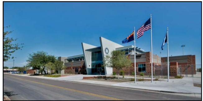
The newly renovated Seattle Mariners' clubhouse is being financed with MDA bonds.
