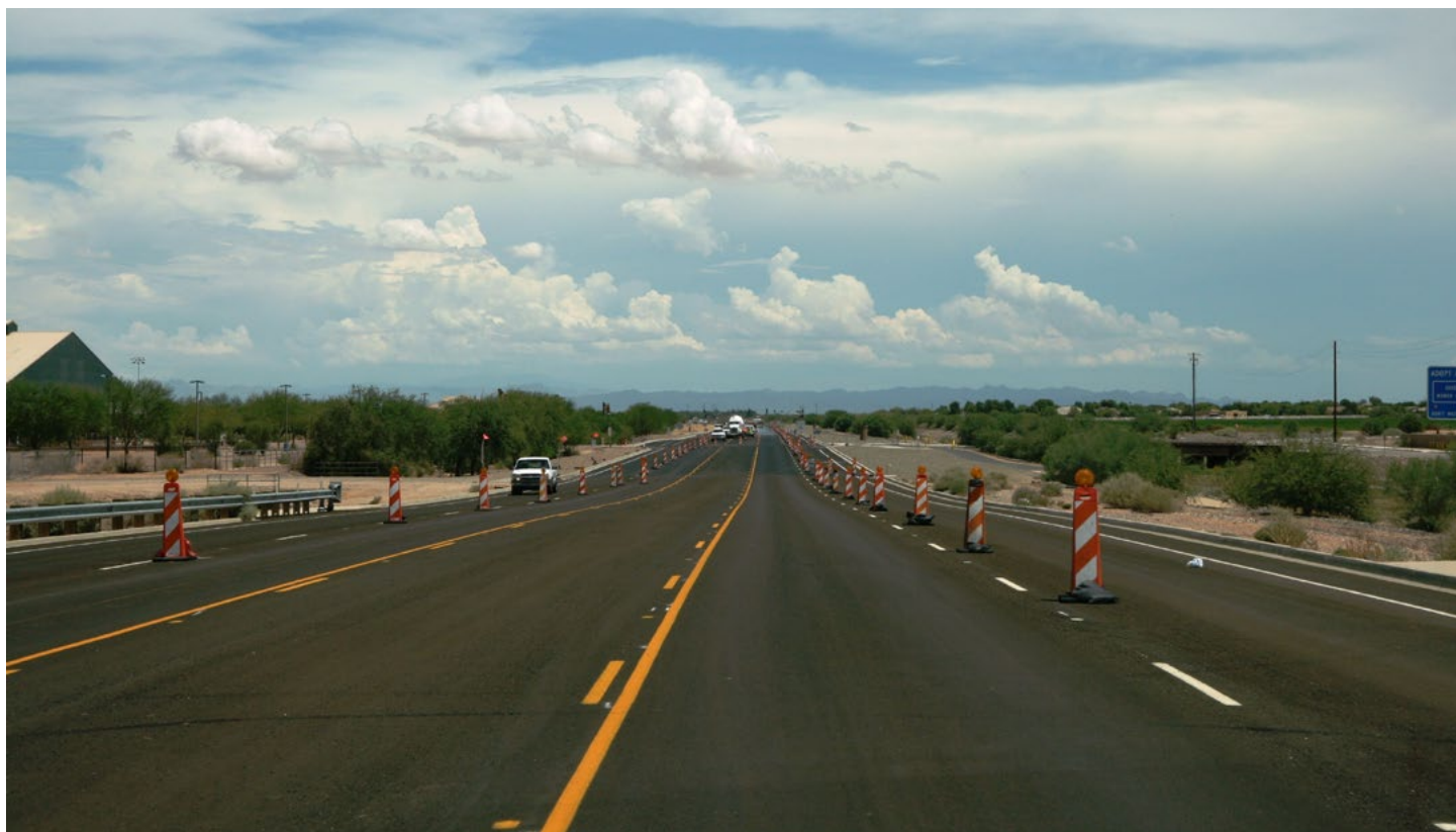
Roadway widening on Riggs Road.
