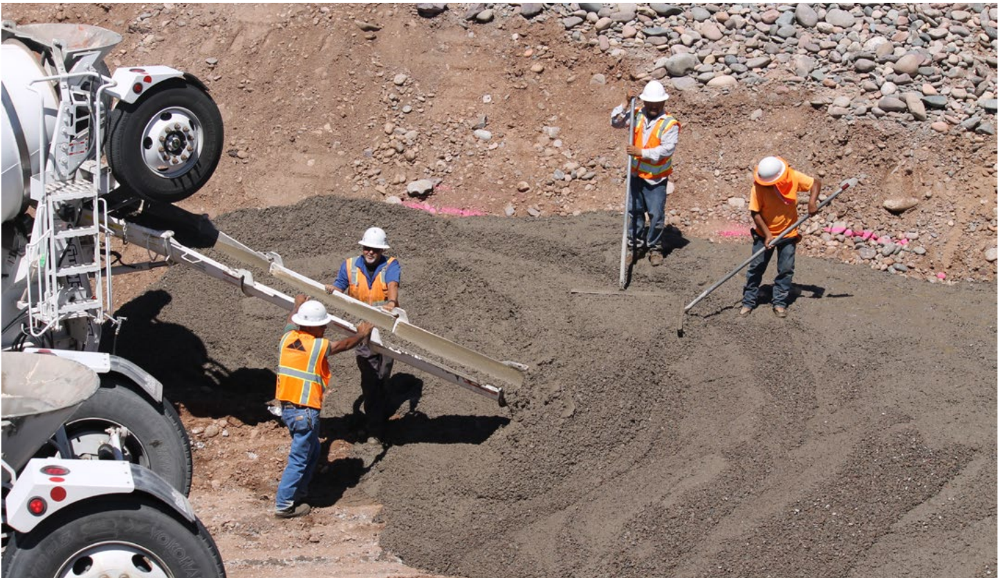
Gilbert Road Bridge repairs.
