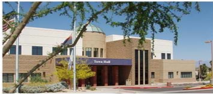
Fountain Hills Town Hall
