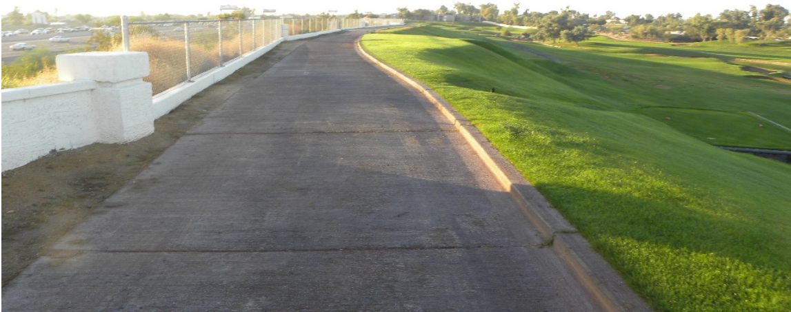
Guadalupe Flood Retarding Structure
