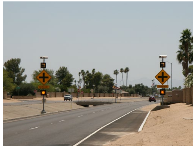
New flashing beacon system at 99th Avenue and Cameo Drive in Sun City
