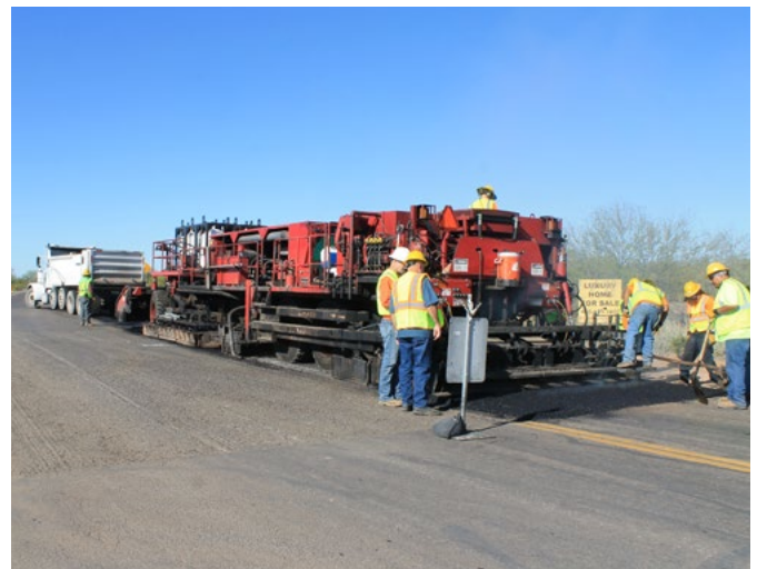
Hot-in-place paving on Patton Road
