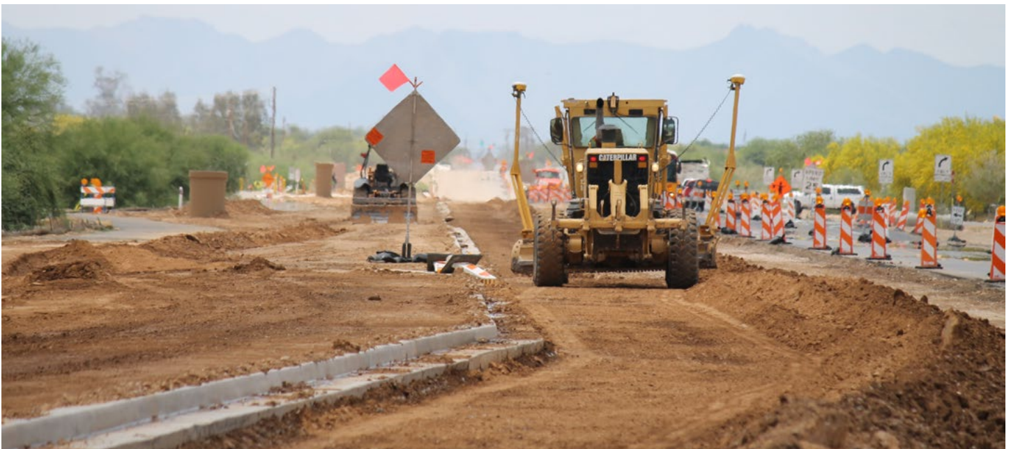
Roadway widening on Riggs Road.
