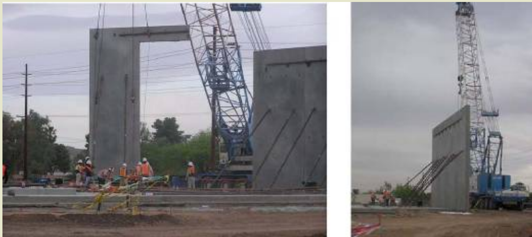
Construction at the McKellips site continues
