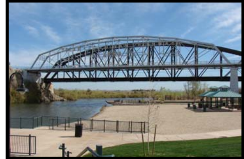
Ocean to Ocean Bridge over the Colorado River.
