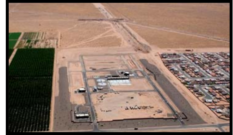
Desert Dunes Water Reclamation Facility
