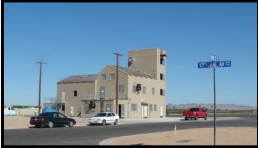
Burn Building located at the City of Yuma Public Safety Training Facility
