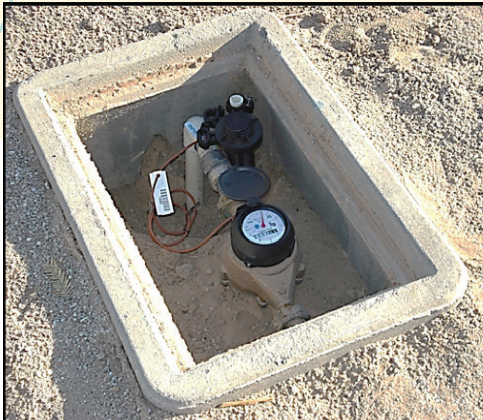
A water meter is fitted with a transmitter to send consumption reading to the meter reader's computer.
