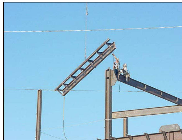
"Setting the Steel" at One City Plaza
