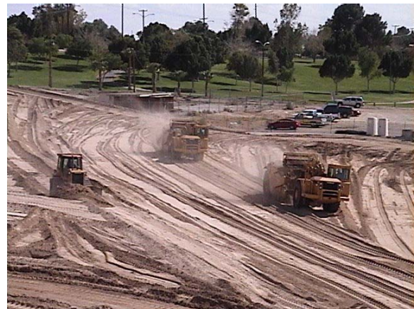
Site grading work begins at Yuma Regional Medical Center
