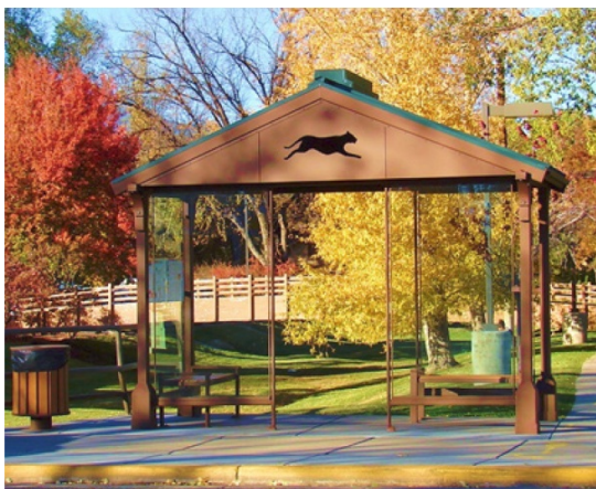
Figure 15: Examples of NAIPTA Bus Shelter
