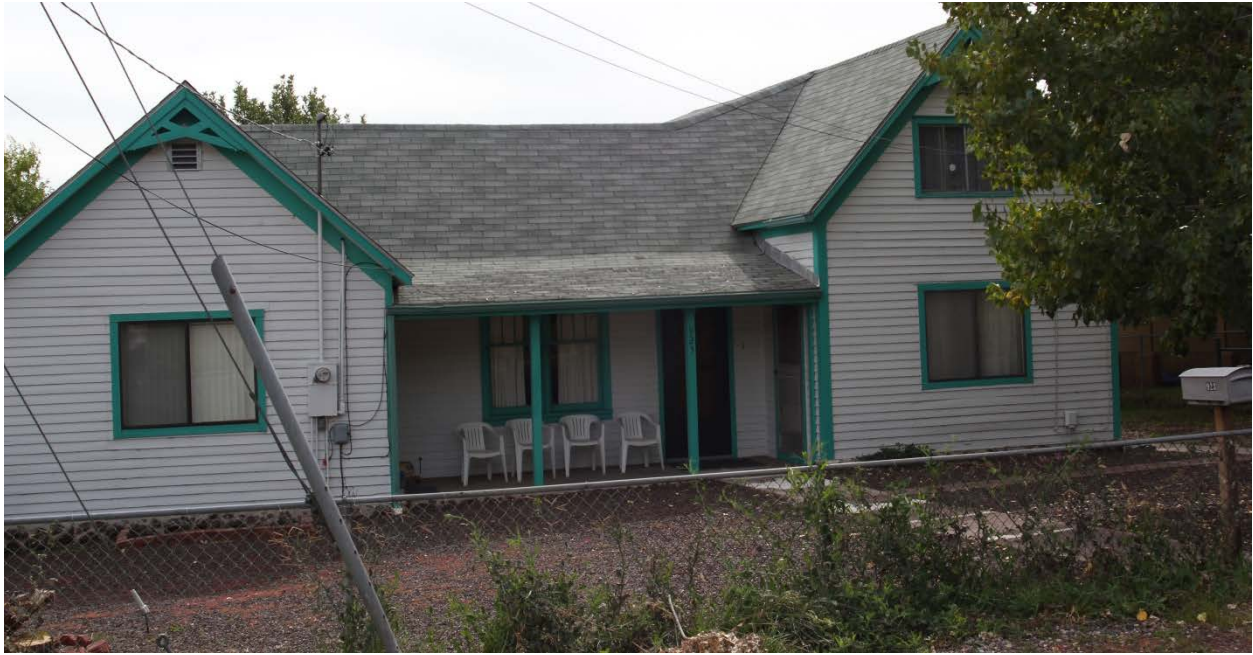
Figure 53: Single-Family Double "L" Home at 923 W. Clay Avenue
