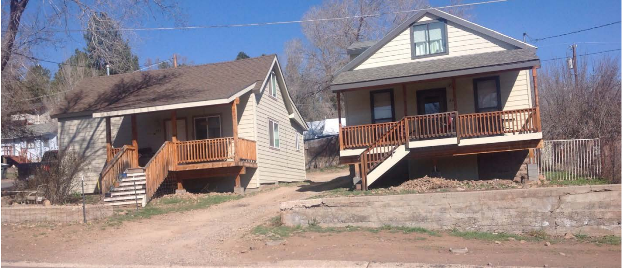
Figure 51: Single-Family Cottages at 829 and 831 W. Coconino Avenue
