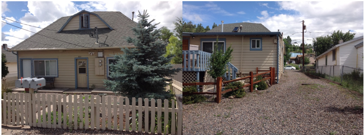
Figure 50: Historic Home Converted to Triplex at 907 W. Clay Avenue (front and back yard views)
