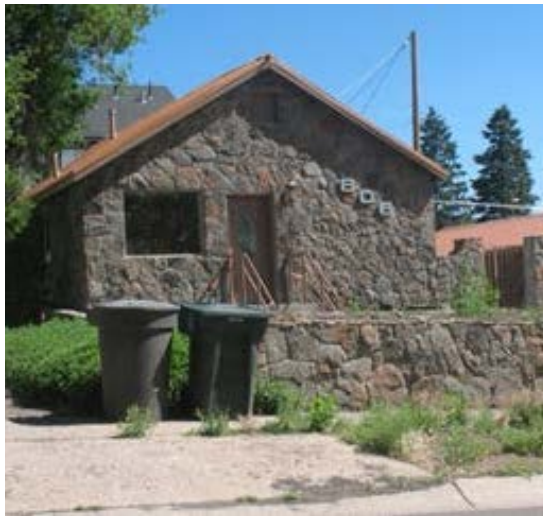
Figure 11: Malpais Facade Typical of Historic Cottages
