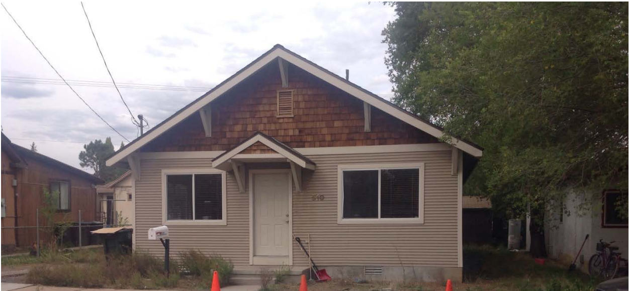
Figure 52: Single-Family Cottage with Covered Stoop at 510 W. Tombstone Avenue
