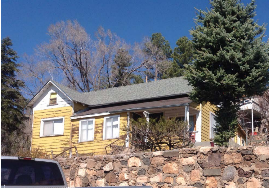
Figure 49: Single-Family “L” Home at 1105 W. Lower Coconino Avenue
