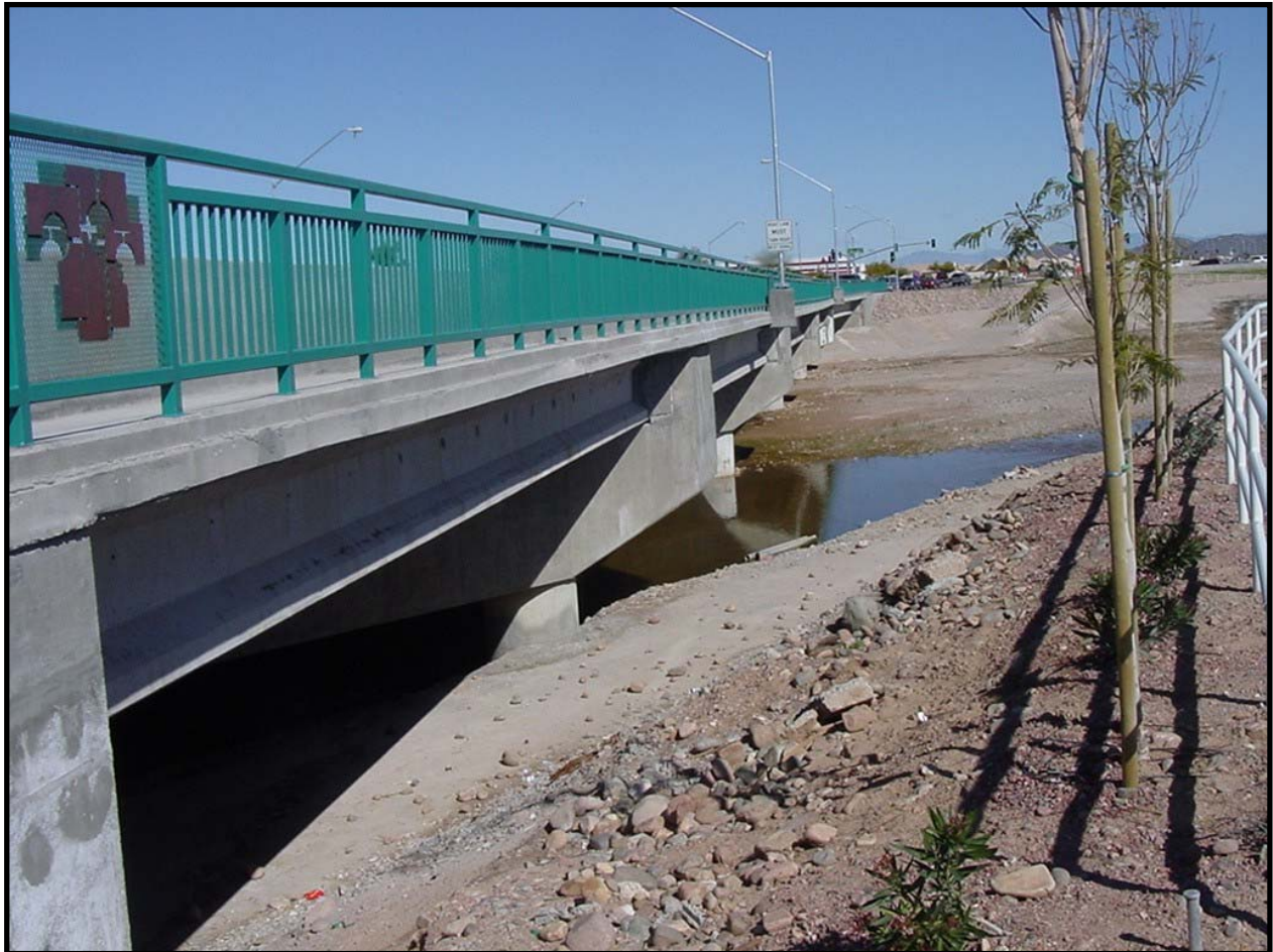
Above: Skunk Creek Rd bridge at 57 th Avenue. Project 8049/80012 Bike & Ped/Skunk Creek @BellRd
