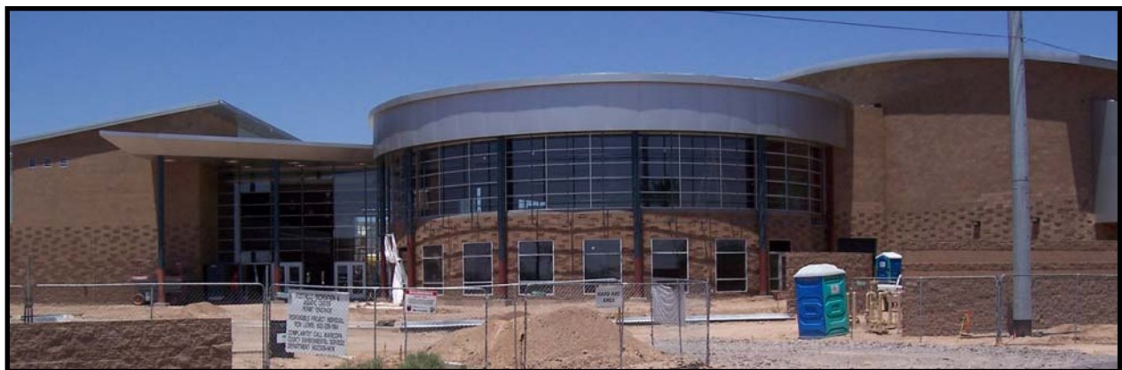
Above: Construction of Foothills Recreation and Aquatic Center at 5600 W. Union Hills Drive is expected to be completed by the end of the summer. Project 8048/70504 Foothills Rec & Aquatics Ctr
