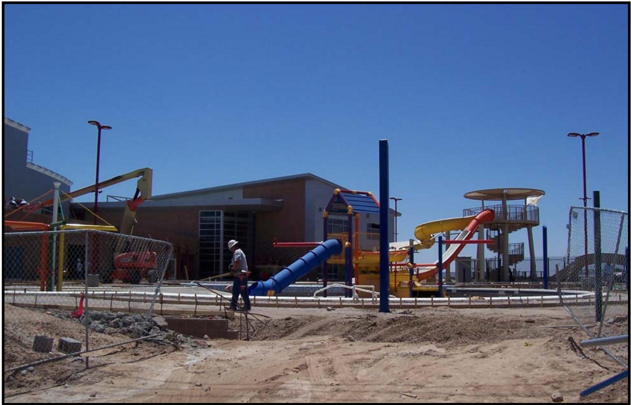
Above: Construction of the Foothills Recreation and Aquatic Center located at 5600 West Union Hills Drive, is scheduled to open in 2006.
