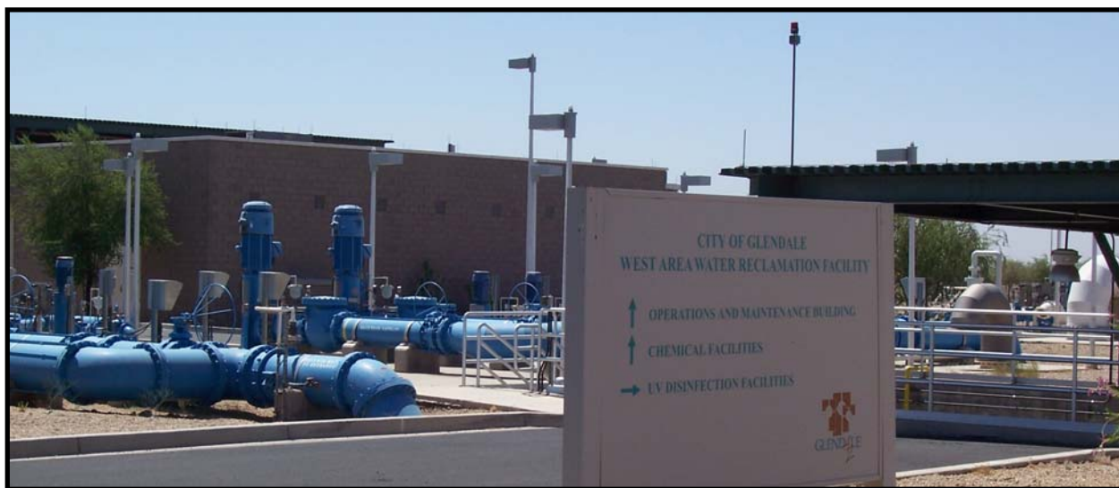
Above: The Western Area Water Reclamation Facility will be expanded to a 10 MGD facility. Project 9246/60003 West Area WWRP.
