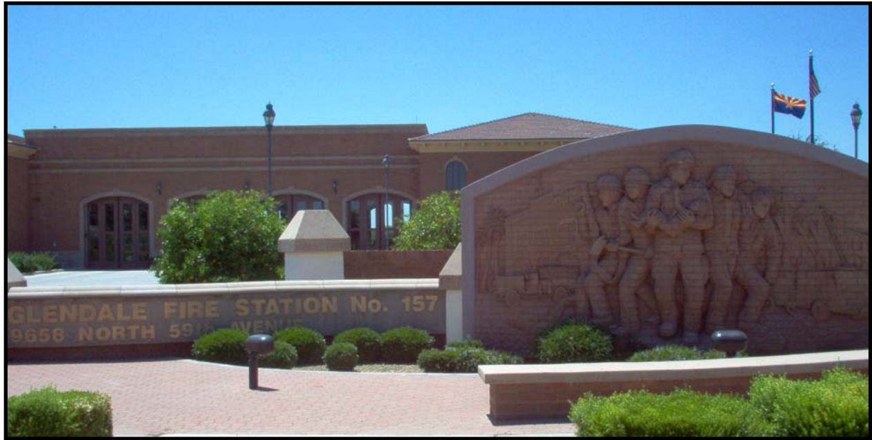
Glendale Fire Station No. 157
