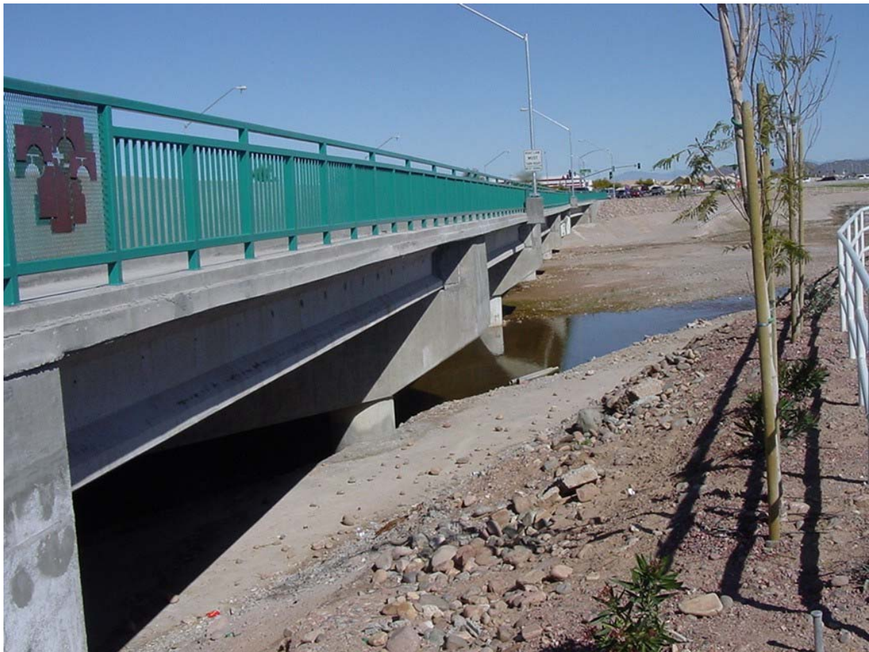
Above: Skunk Creek Rd bridge at 57 th Ave.
