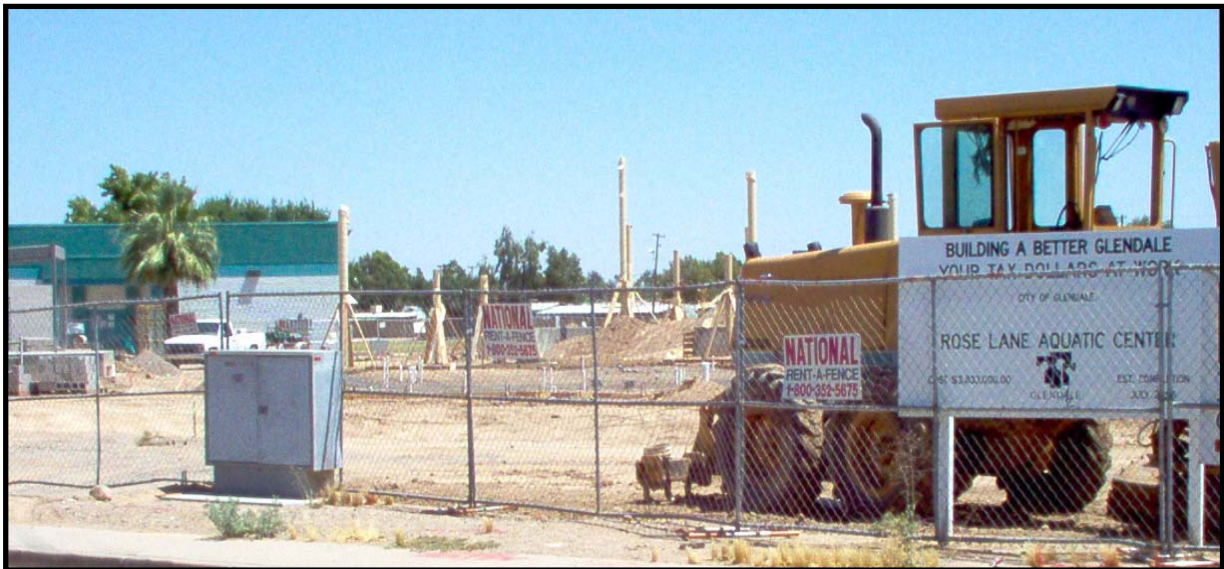
Above: Construction of the Rose Lane Aquatic Center located near 51 st Avenue and Marlette Avenue, south of Glendale. The aquatic center is scheduled to open mid summer 2005.
