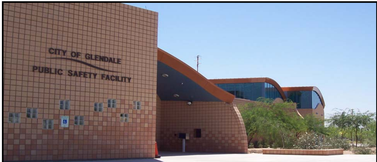
Above: The newest public safety facility to the City of Glendale is both a Police and Fire station. It is located on 83 rd Ave South of Glendale Ave.
