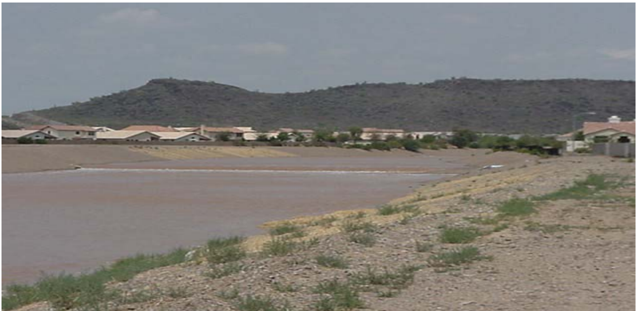
Above: Skunk Creek – West of 51 st Avenue Alignment.
