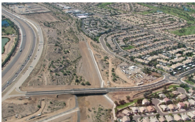
Federal dollars paid for much of the Beardsley Road Connector project , which provided enhanced freeway access for residents living in the northern reaches of Peoria.
