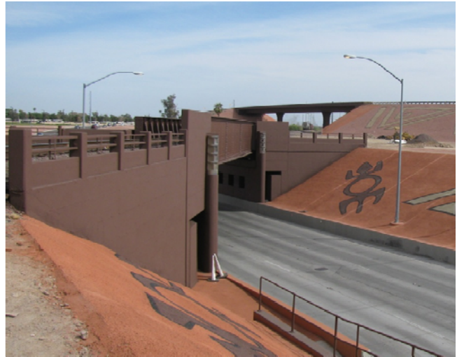
ADOT installed the first land form graphics in Peoria as part of its Grand Avenue Improvements.
