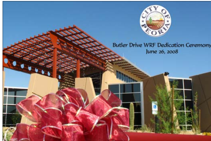
Revenue bonds helped pay for the Butler Drive Wastewater Reclamation Facility, the city's largest ever capital project.
