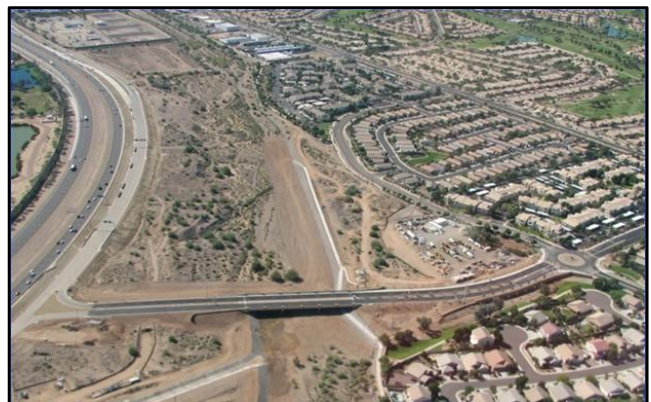
Federal dollars paid for much of the Beardsley Road Connector project, which provides enhanced freeway access for residents living in the northern reaches of Peoria.
