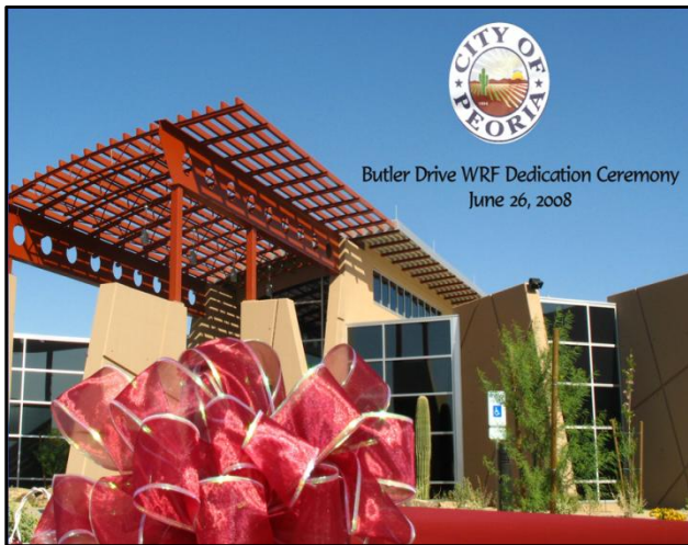
Revenue bonds helped pay for the Butler Drive Wastewater Reclamation Facility, the city's largest ever capital project.
