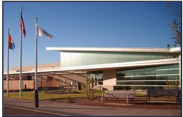
The Community Center in Old Town Peoria was recently remodeled and expanded.
