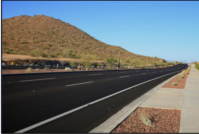
The city was reimbursed almost $21 million for its Happy Valley Road project through Maricopa County's Arterial Life Cycle Program.
