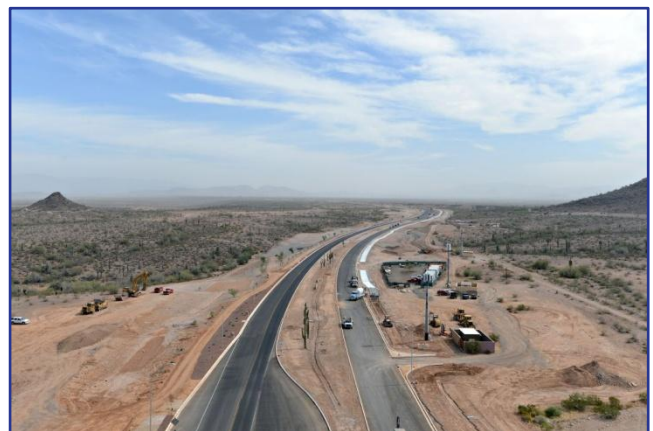
Construction is nearing completion on Lake Pleasant Parkway in northern Peoria.
