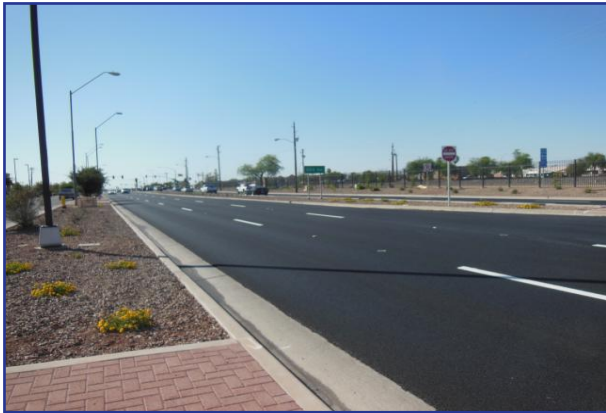
The city recently widened 83 rd Avenue to four lanes adjacent to the new Pioneer Community Park.
