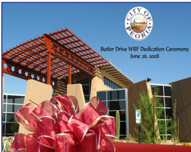
Revenue bonds helped pay for the Butler Drive Wastewater Reclamation Facility, the city's largest ever capital project.
