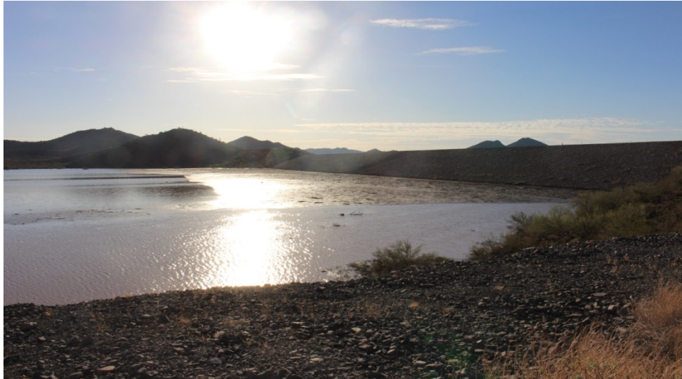
New River Dam
