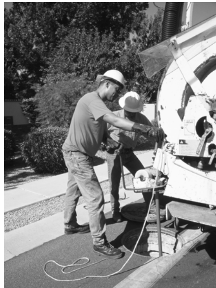
Crew at work on waterline
