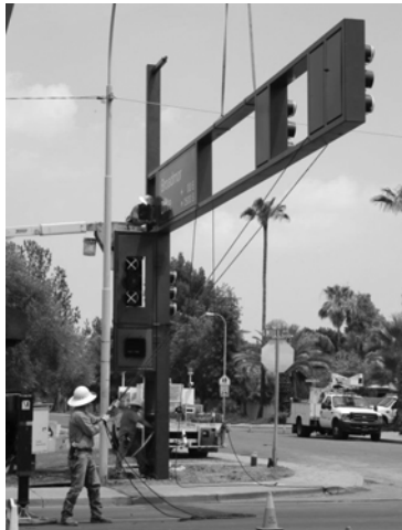
Traffic signal under construction
