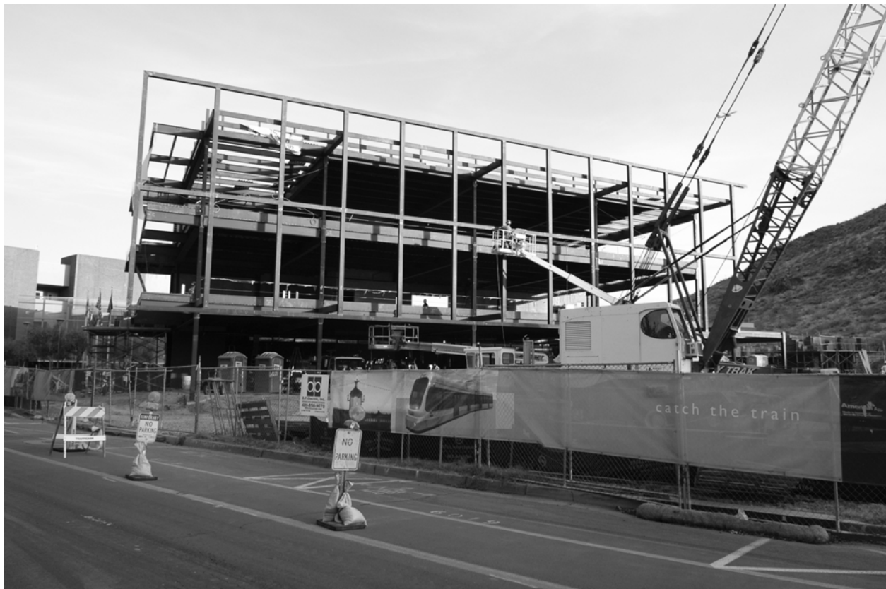
Tempe Transit Center under construction
