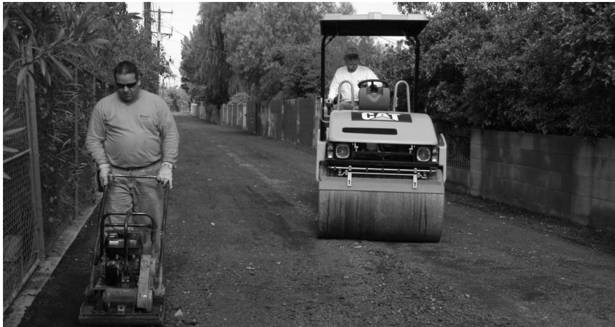
Alley improvements in progress
