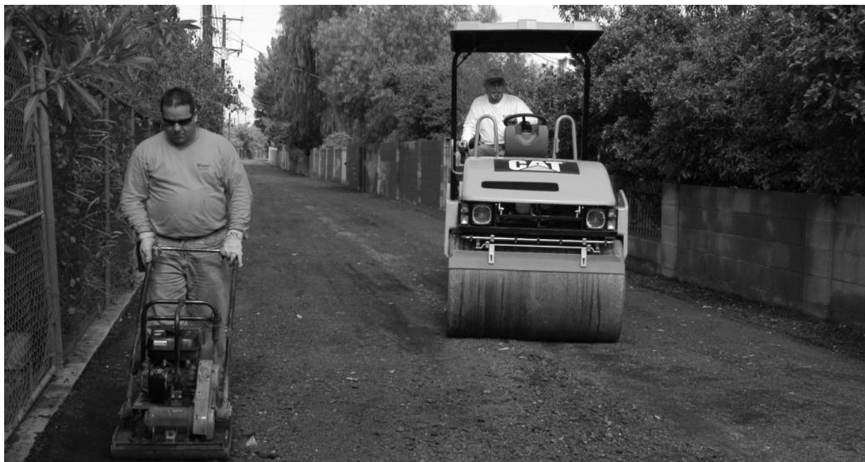
Alley improvements in progress
