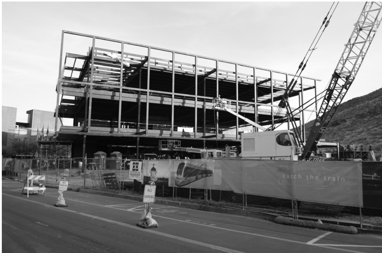
Construction of the Tempe Transportation Center
