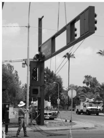
Traffic signal under construction
