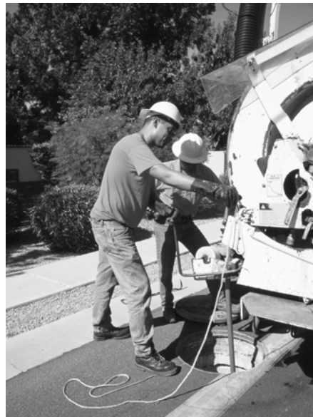
Crew at work on waterline
