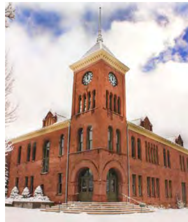
Coconino County Courthouse - December 2012
