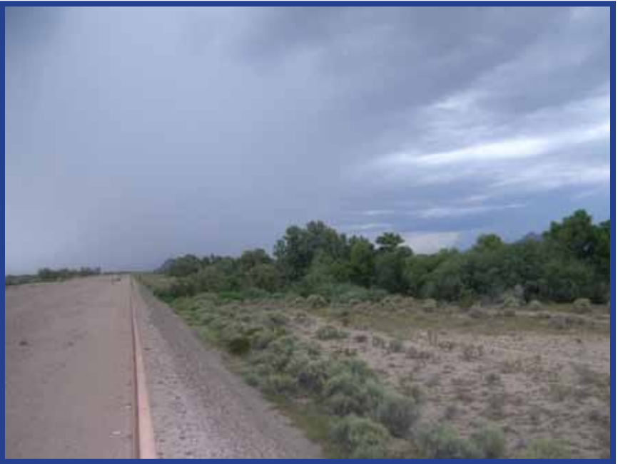
Lower Santa Cruz Levee
